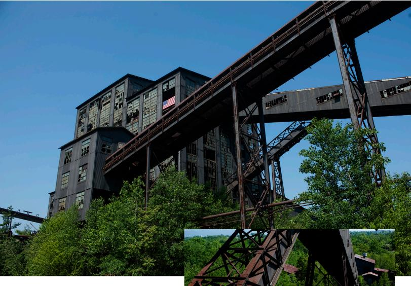
Built in 1939 atop the bones of the earlier Maxwell Breaker (1895-1938), the Huber Breaker in Ashley, PA is the largest and last of its kind. A breaker, simply put, is a giant machine built to look like a building, that smashes large chunks of coal into smaller, usable chunks of coal. The Huber Breaker closed in 1976, and was abandoned in 1978.
